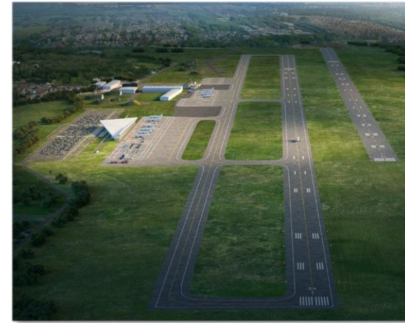
Bird's eye view of the airside development plan (Source: database of the Municipality of Debrecen)
